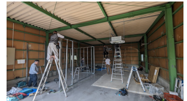
Construction on new building
